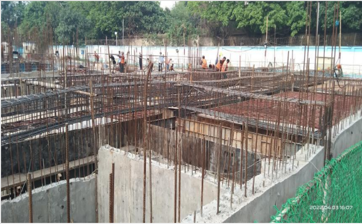
GF slab work progress on 03-04-22
