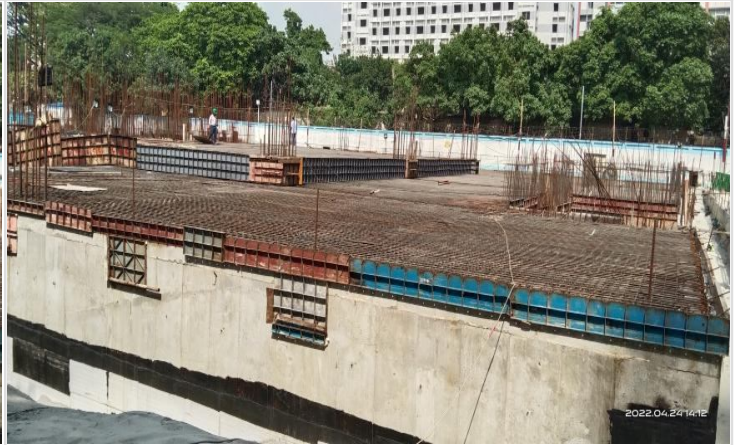
Slab inspection on 23-04-22
