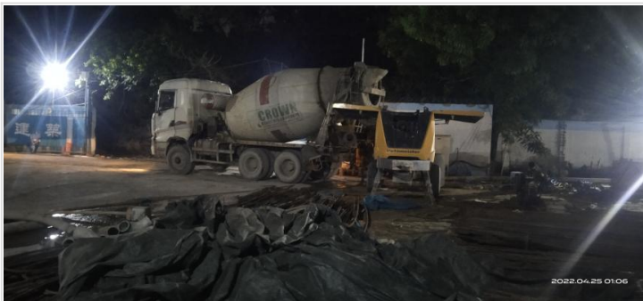
Ready mix Concrete Truck
