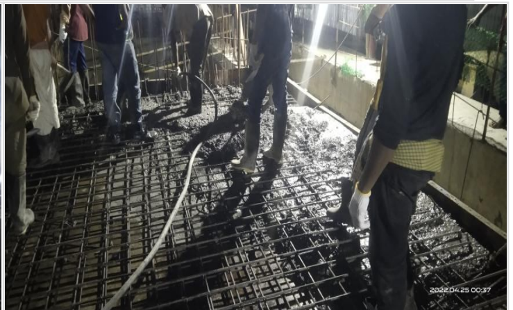
Ground Floor Slab concreting on 24-04-22
