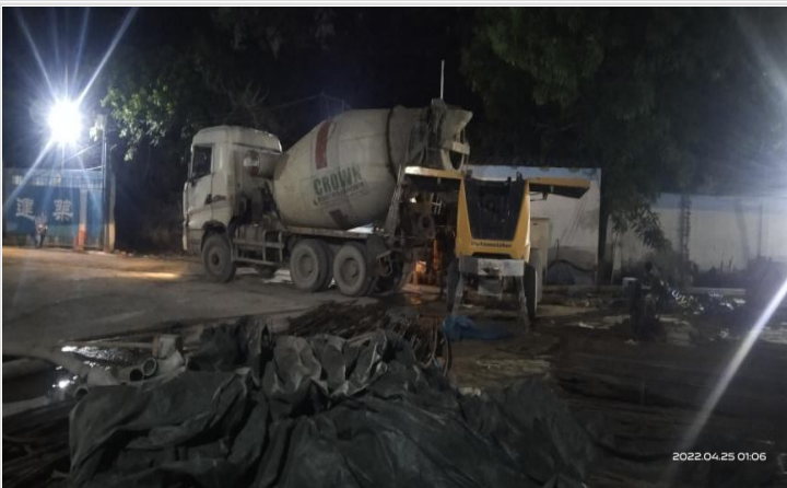
Ready mix Concrete Truck on 24-04-22
