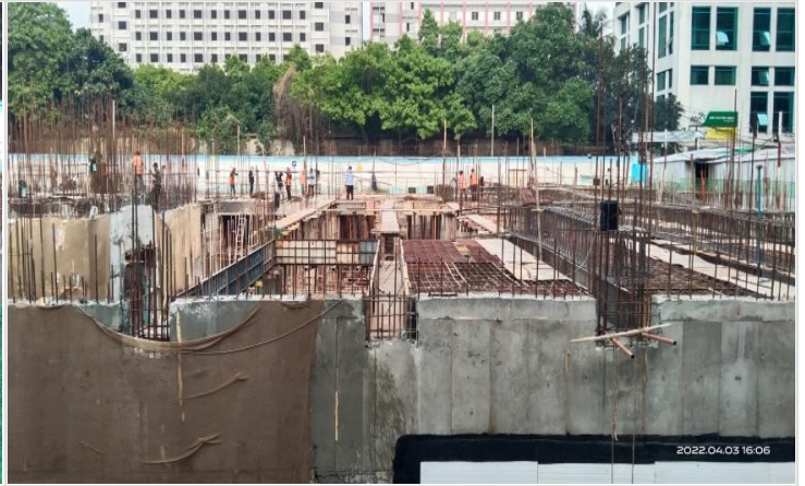
Work progress on 03-04-22
