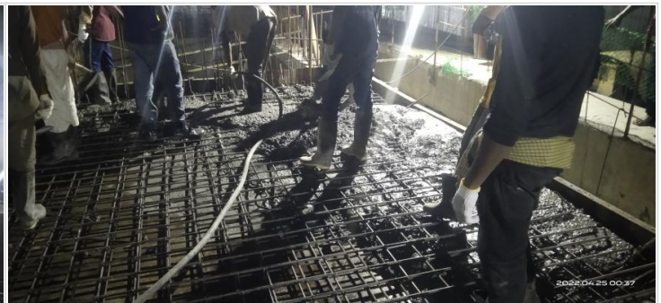
Ground Floor Slab concreting
